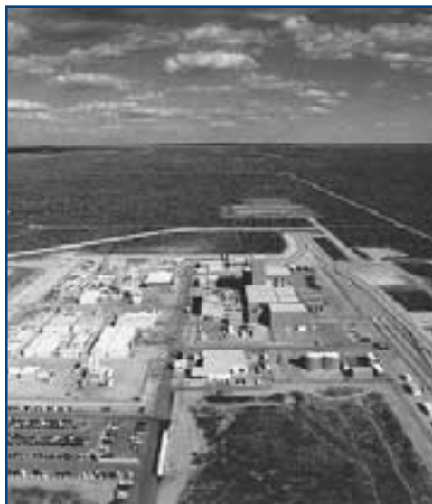
Figure 23. Aerial view of the WIPP
